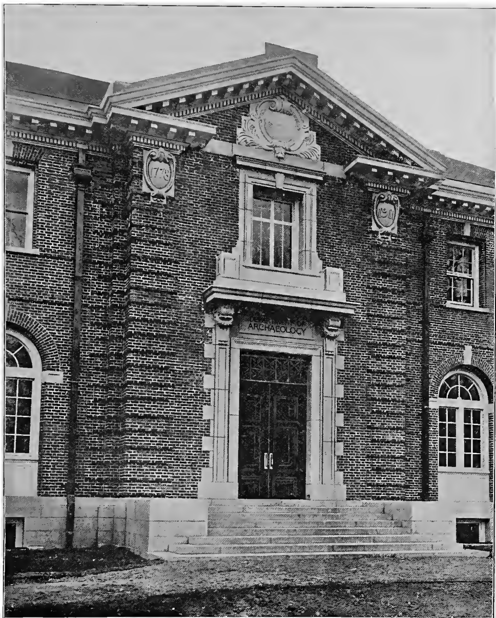
FIG. 3 — DETAIL OF THE FRONT OF THE ARCHAEOLOGY BUILDING
